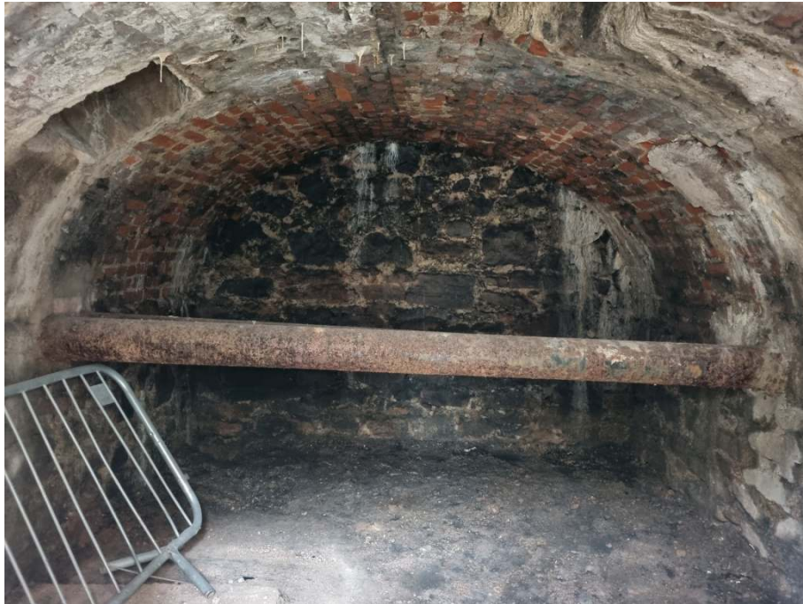
Plate 5: arched basement with heating pipe extending across it.
