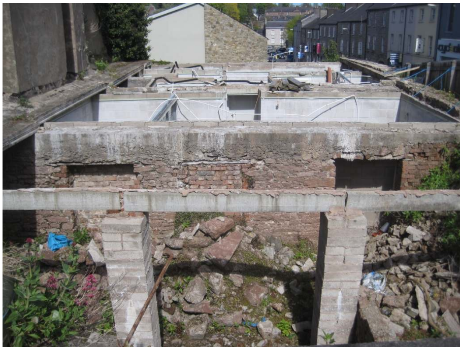
Plate 2: rear wall of basement area showing bricked up openings and modern construction beyond.
